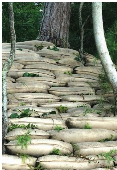
EnviroLok bags were placed on the eroded slope and native shrubs, wildflowers, grasses and groundcovers were planted in between the bags, where they will root and stabilize the ground.
